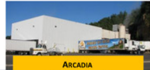
ARCADIA PROCESSING PLANT
